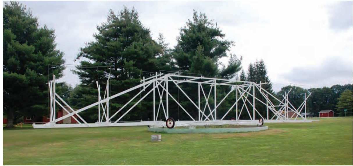
This reconstruction of Karl Jansky's first radio telescope was built on the grounds of the National Radio Astronomy Observatory in Green Bank, West Virginia. Jarek Tuszynski
