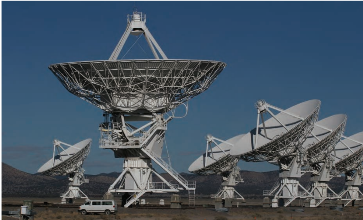
These 82-feet-in-diameter (25 m) radio antennae make up the Very Large Array (VLA) radio astronomy observatory in New Mexico. Data from the 27-dish antennae is combined, making it an overall 22-mile-wide (36 km) radio telescope. Tom Uhlman Photography
